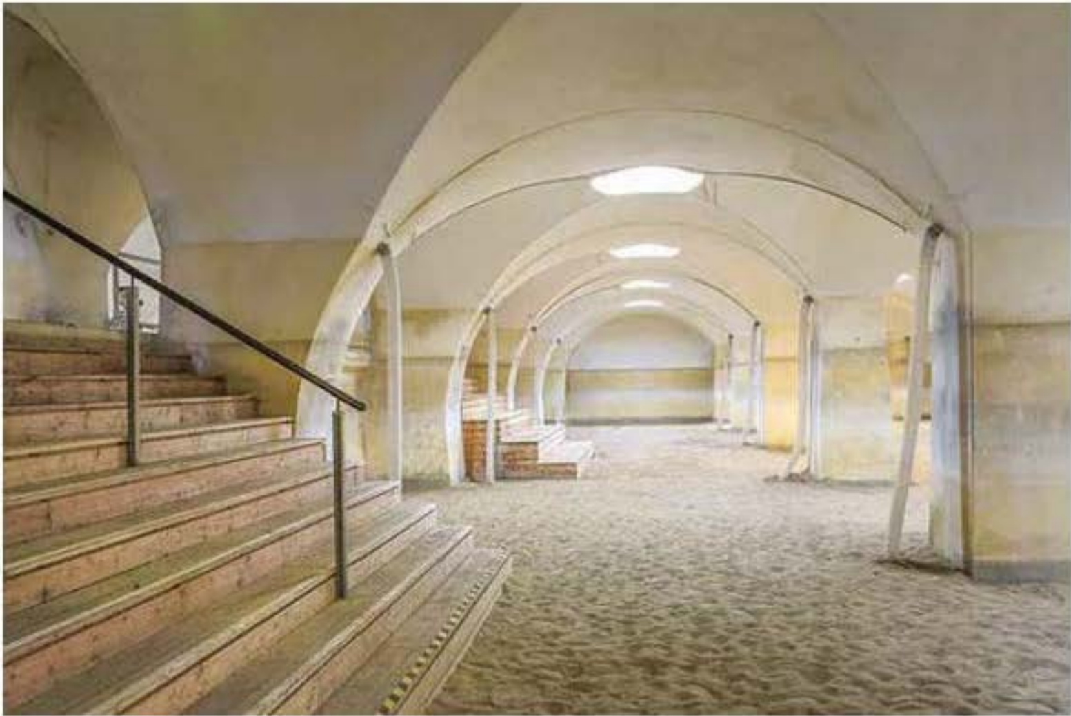
Water filter building. Base © Johanna Keimeyer
